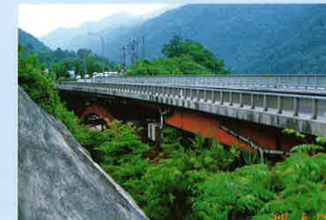
Arch part: LUMIFLON® Closer part: Alkyd
