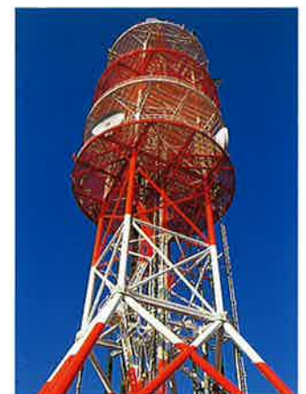
Name: NTT Sekimoku Network Center LUMIFLON®: Solvent Substrate: Iron
