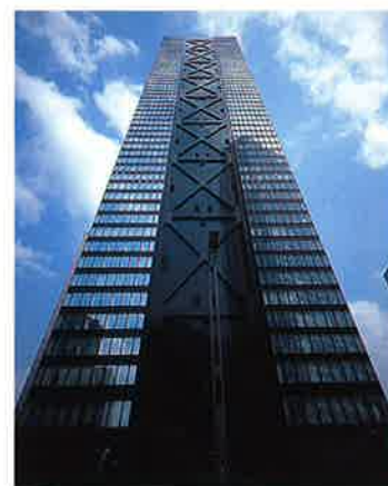
Name: Shinjyuku Mitsui Building LUMIFLON®: Solvent Substrate: Aluminum
